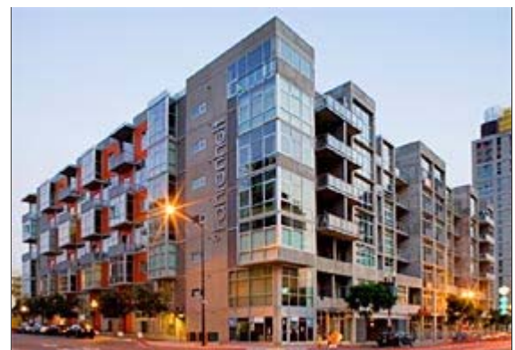
MIKE TORREY PHOTOGRAPHY – miketorrey.com ORCHID FOR ARCHITECTURE: "This is the type of innovation we need from developers," jurors said of Fahrenheit. Studio E Architects designed the live/work spaces to wrap around a parking structure.
